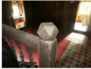
Figure 6: Geometrical head shaped at handrail of stairs to attic Source: USIM, 2018
